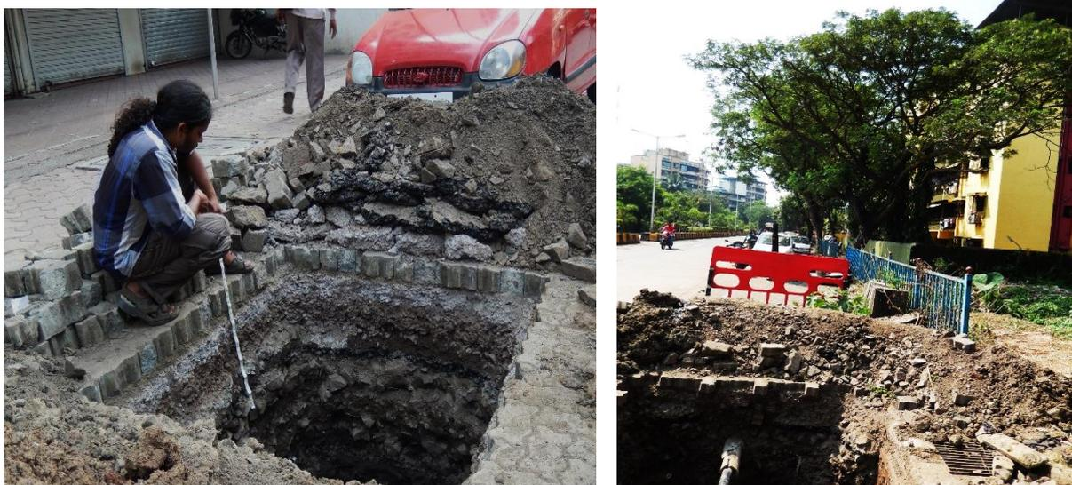
***Bases and vicinities of the trees were dug to find out the thickness of the soil layer below ground. Construction material was found in place of soil and organic content.***
